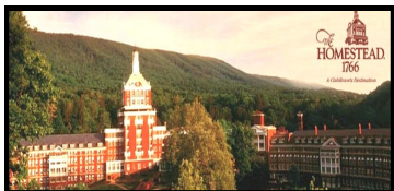
The Homestead, Hot Springs, VA
